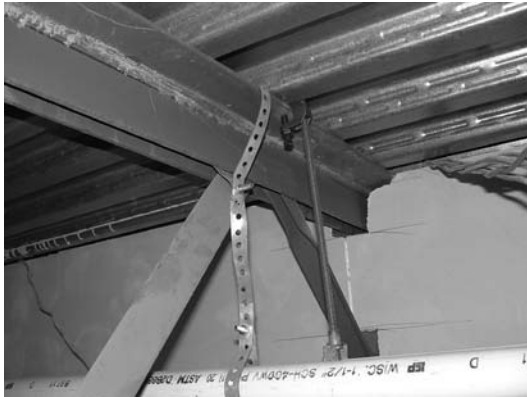
Fig. 7. Joist with crimped web members.
