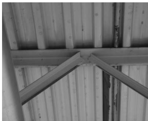
Fig. 5. Angles interfering with top chord reinforcement.
