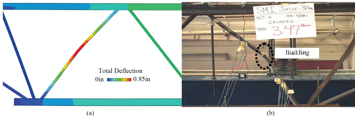
Figure 12: Flexural buckling of 30 in. deep joist diagonal at failure. (a) Model (b) Yost et al. (2006)
