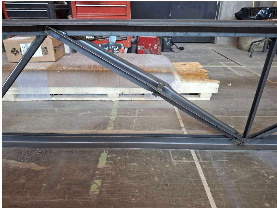
Figure 16. Typical failure mode for specimen group B2 (specimen B2a shown)
