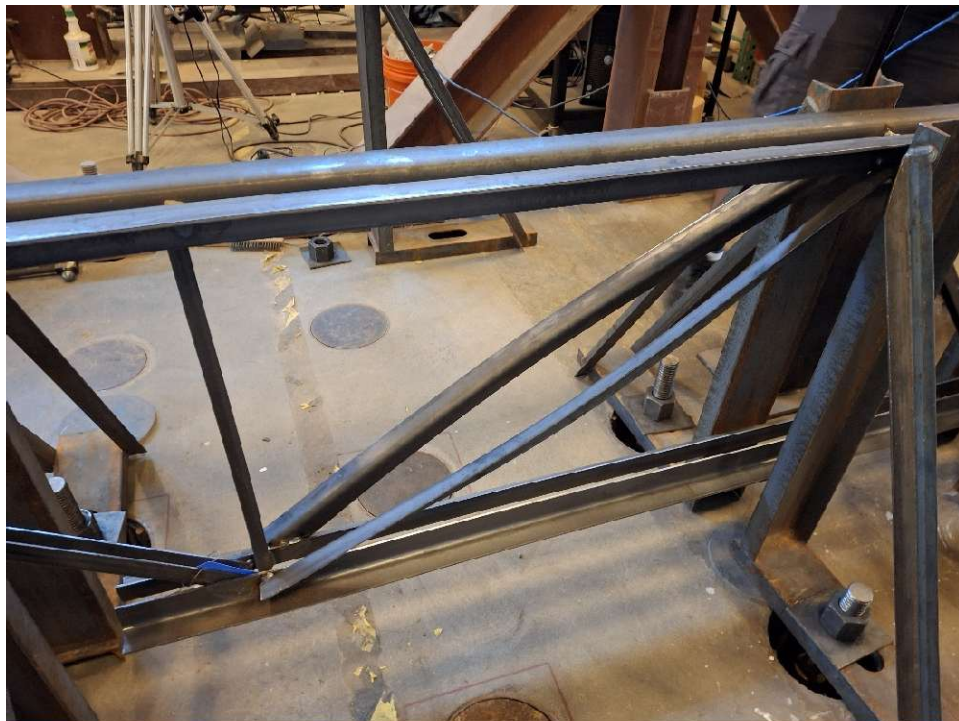
Figure 14. Typical failure mode for specimen group B0 (specimen B0c shown)
