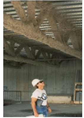
Figure 16. Spray-applied fireproofing on a CJ-Series joist.
