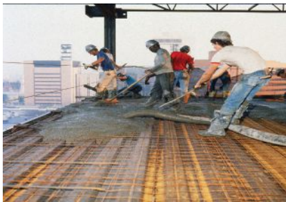
Figure 13. Concrete is pumped over the steel deck and supporting steel joists.
