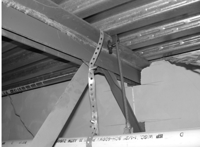
Joist with Crimped Web Members
