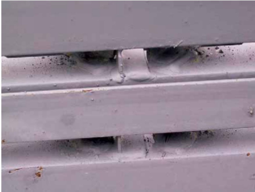
Cold-Rolled Channel Webs Welded to Bottom Chord
