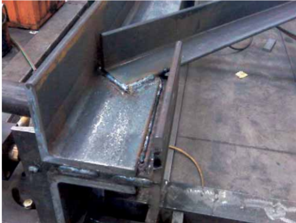
Lapped Seat Angle to Top Chord Fillet Welds
