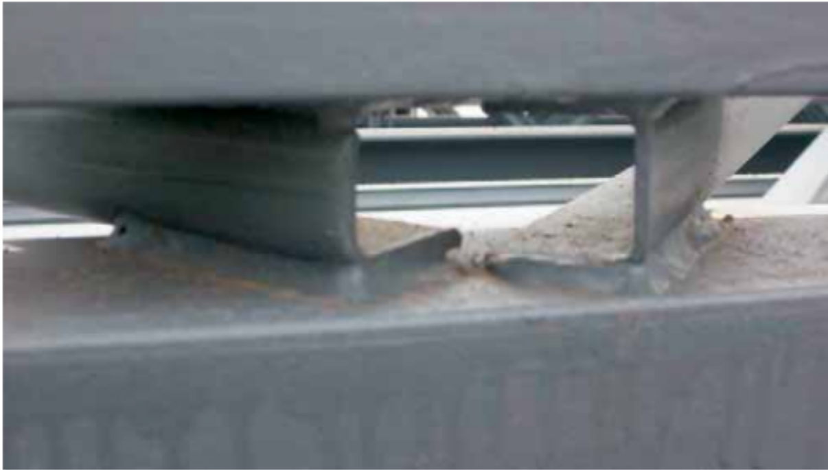
Cold-Rolled Channel Webs Welded to Top Chord
