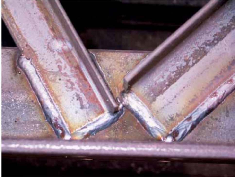
Fillet Welded Double-Angle Web Members to Top Chord
