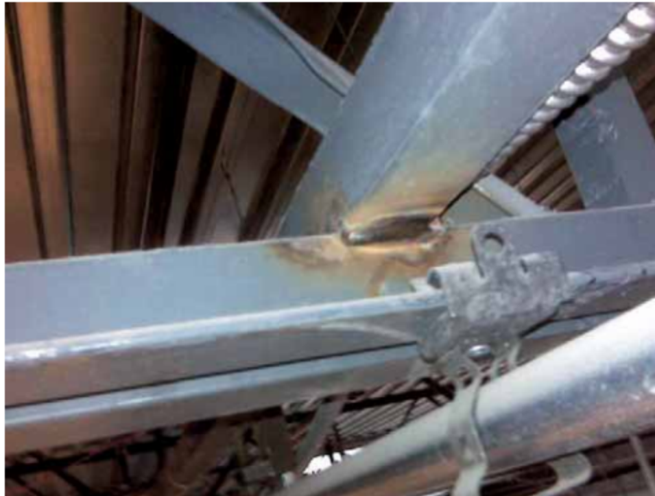
Acceptable Weld of Bridging Angle to Bottom Chord
