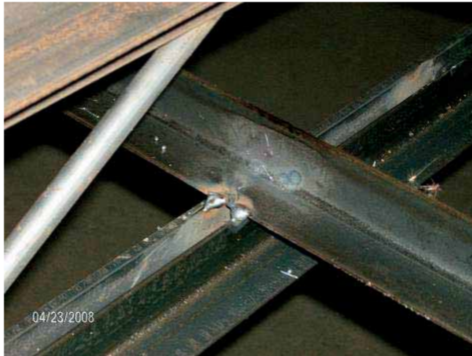
Unacceptable Weld of Bridging Angle to Bottom Chord
